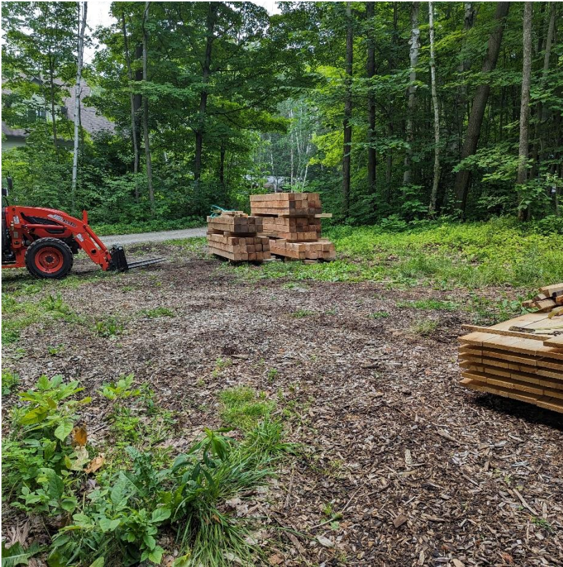
Clearing, facing south.
