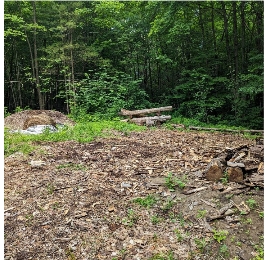
Clearing, facing north.
