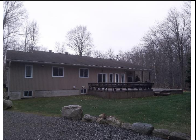
IMAGE 14 HOUSE, DRIVEWAY AND LAWN AREA
