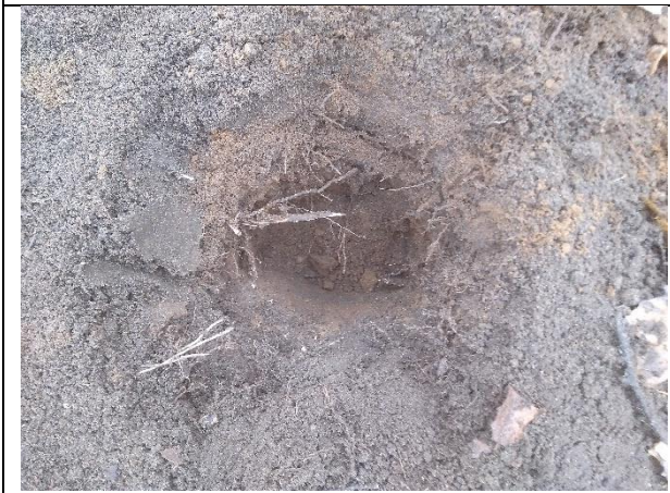
IMAGE 11 COMPLETED TEST PIT
