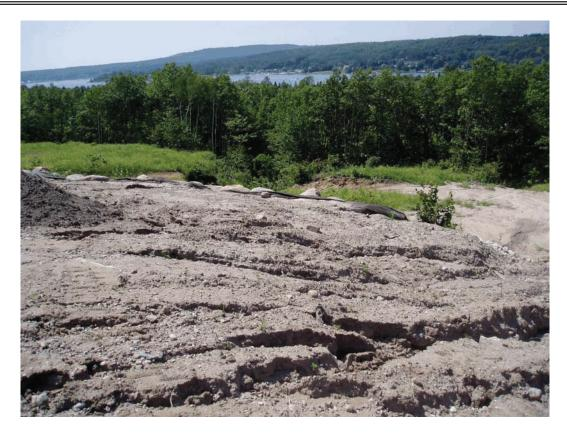
Photograph 9. Construction activity to southeast of property, showing erosion and sediment released towards property (August 9, 2010).
