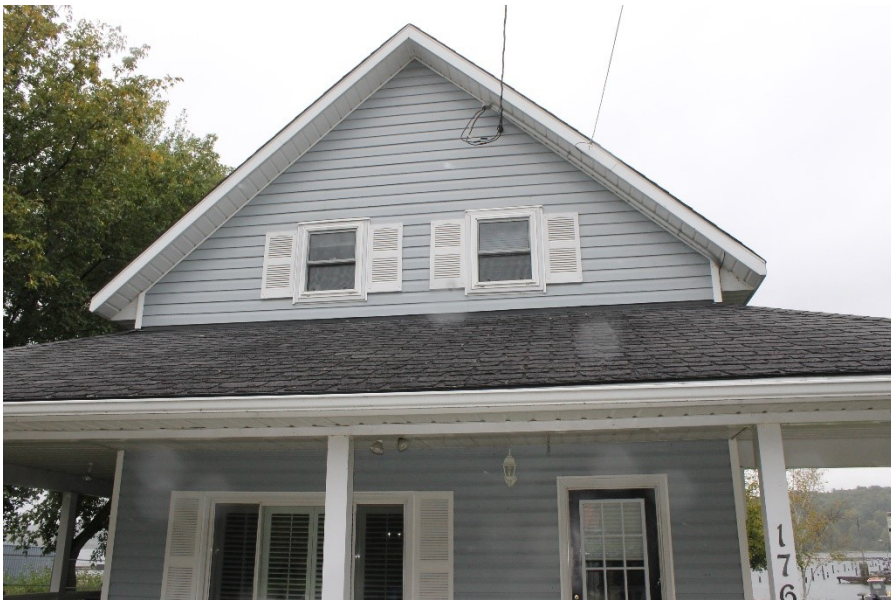
Photograph 8. Exterior of residential dwelling at the south end of the property. (September 25, 2018)
