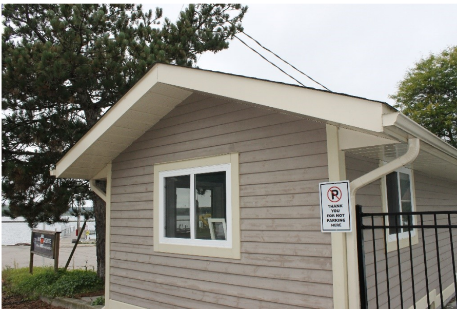
Photograph 6. Exterior of small motel structure central area of the property. (September 25, 2018)
