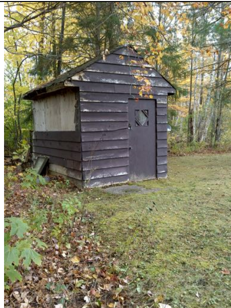
Image 20 Existing Structure – Shed
