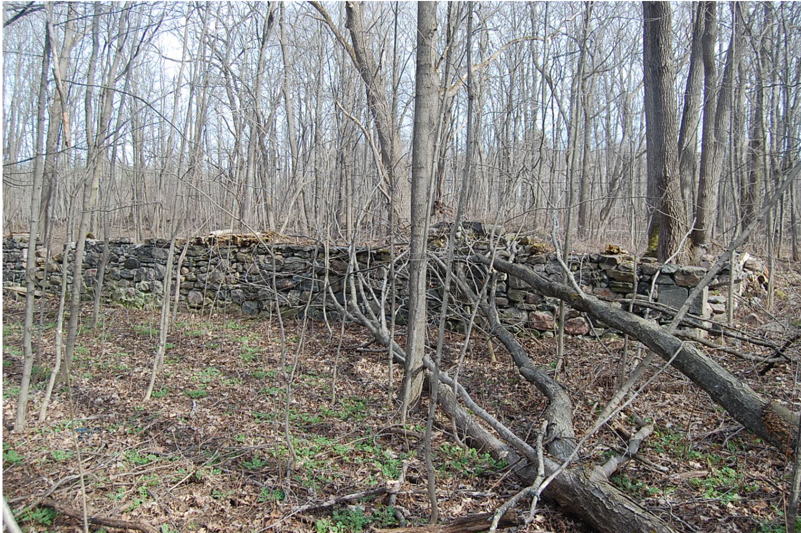
Photo 8 - North face of remnant stone foundation on east edge of Lot 5
